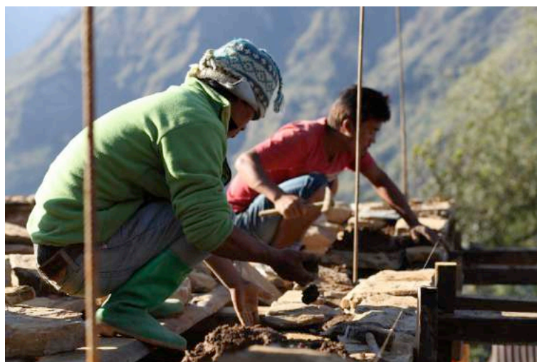
Figure 1 Construction à Yamgaon
